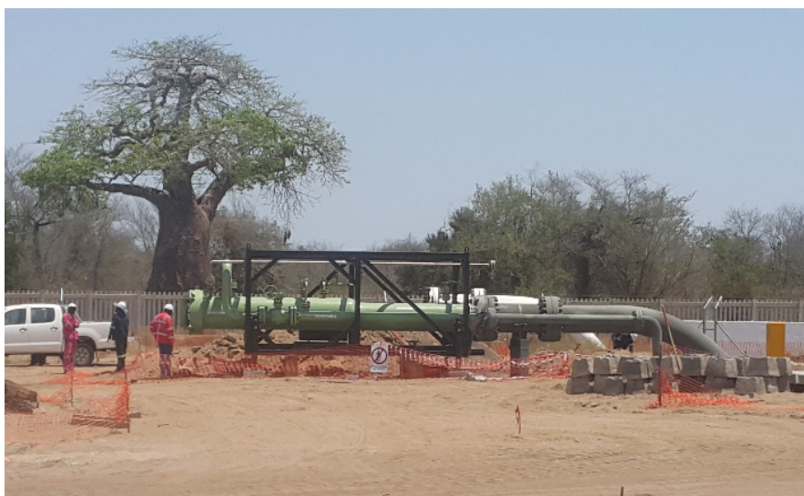
Figure 7: Example of a pigging station (Photo from Mr N Ephraim, iGas).
