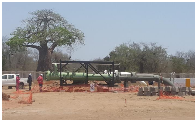
14 15 Figure 4: Example of a pigging station (Photo from Mr N Ephraim, iGas).
