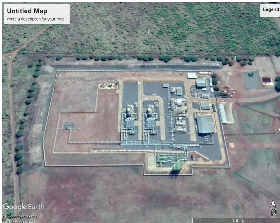
Figure 1: Example of a compressor station – Location: Komatipoort (Source: Google Earth)
